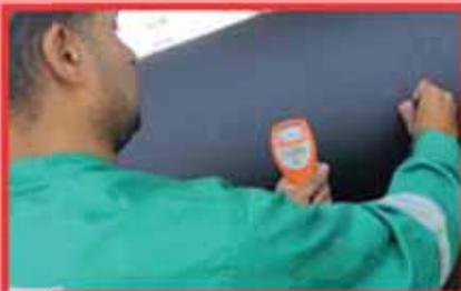
BITUMEN COATING THICKNESS
